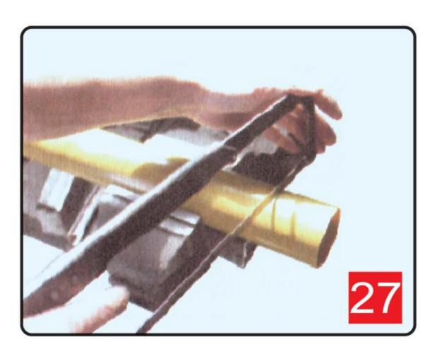
4. Shorten the plastic shield tubes one at a time by cutting the same length that was cut from the inside drive tubes.
